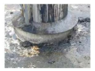
FiberTite roof still performing after decades of exposure to grease and acids from this food processing plant's roof mounted mechanical units.
